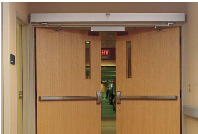
Two examples of Fire Doors in a commercial building and an academic building.
