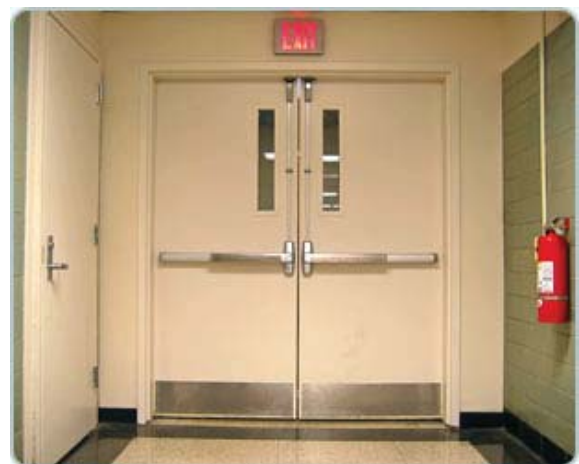
Two examples of Fire Doors in a commercial building and an academic building.
